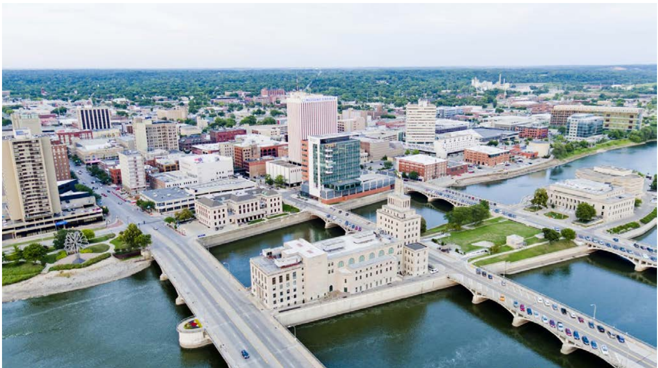
Downtown Cedar Rapids looking east into the Lower Cedar Watershed
