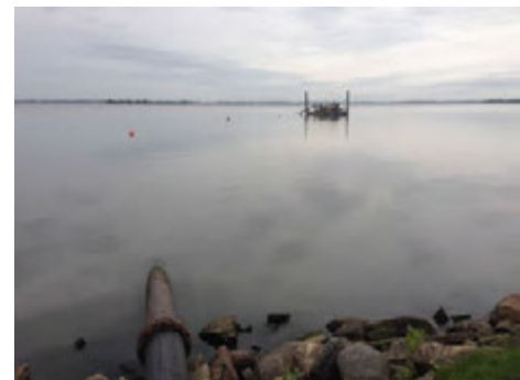
Storm Lake Dredging Operation
