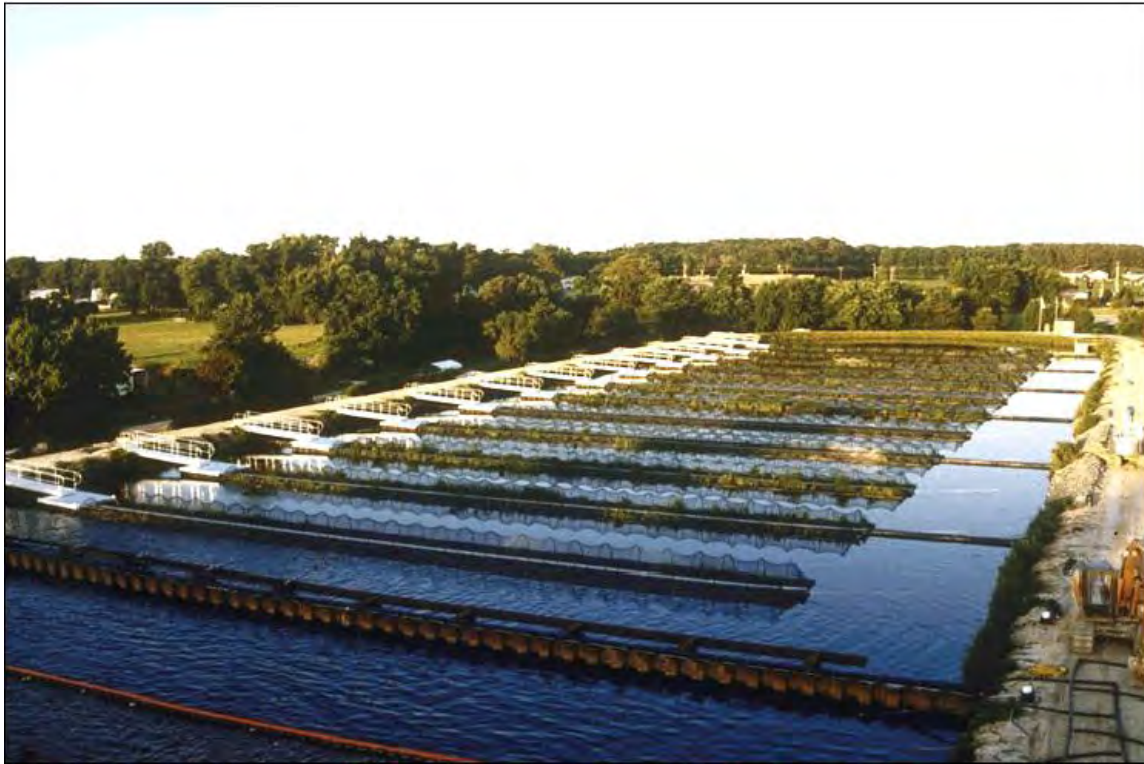
Tyson Restorer-based treatment system, Berlin, Maryland
